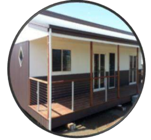
Roofing, Gutters & Fascia Colorbond Corrugated Iron
