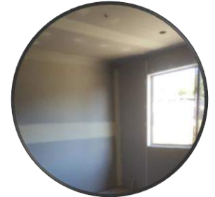
Internal Lining Plastered gyprock walls and ceiling (Villaboard walls in wet areas)
