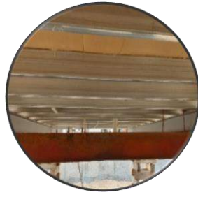
Base Frame Steel Joist & Bearers
