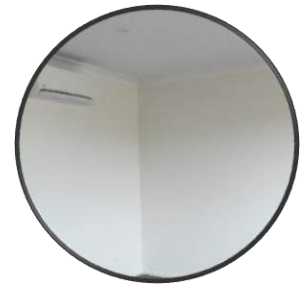
Paint Dulux Wash & Wear- 3 coat system
